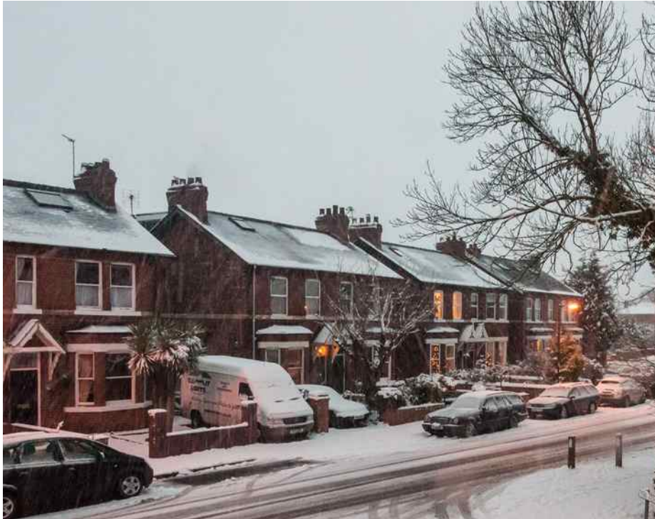
Former Railway Housing
