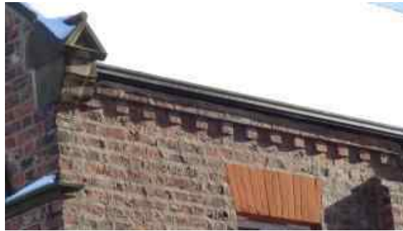
Decorative Banding and Brick Cambered Lintel
