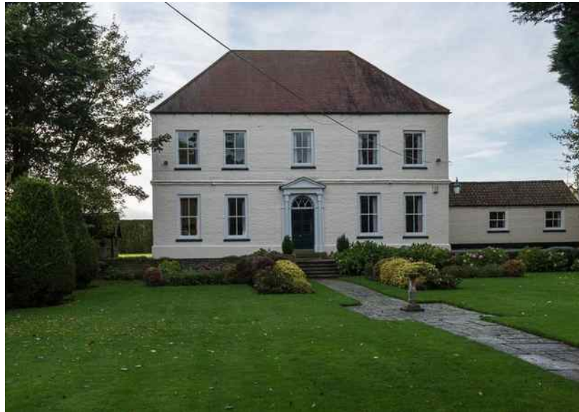
Manor House Farmhouse, Strensall
