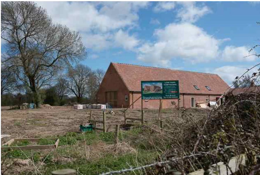
Towthorpe - The conversion of agricultural buildings
