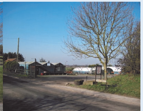
Disused nursery buildings.
