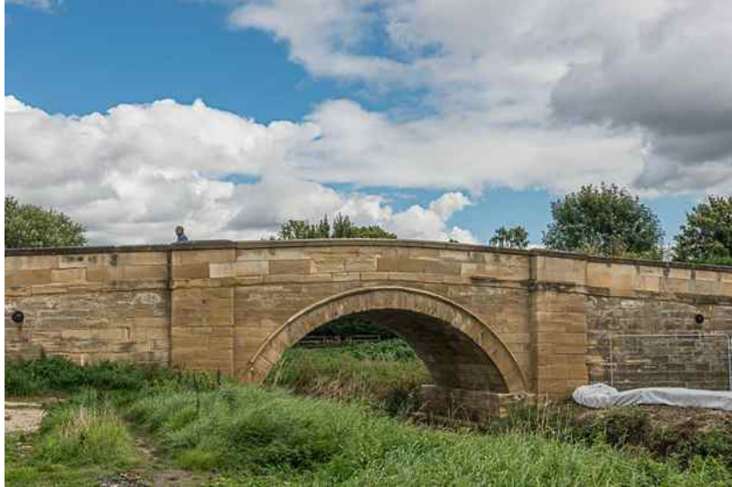
Strensall Bridge - John Carr's Bridge
